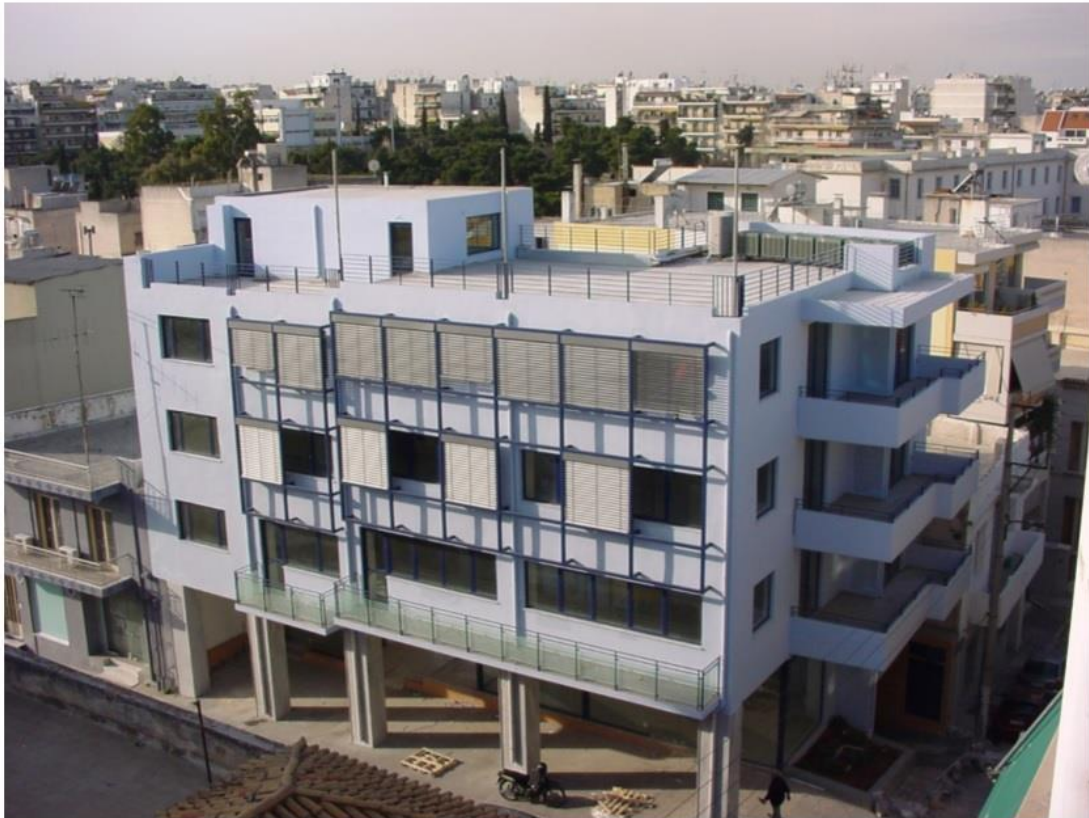
Photo 1: General view of the building
